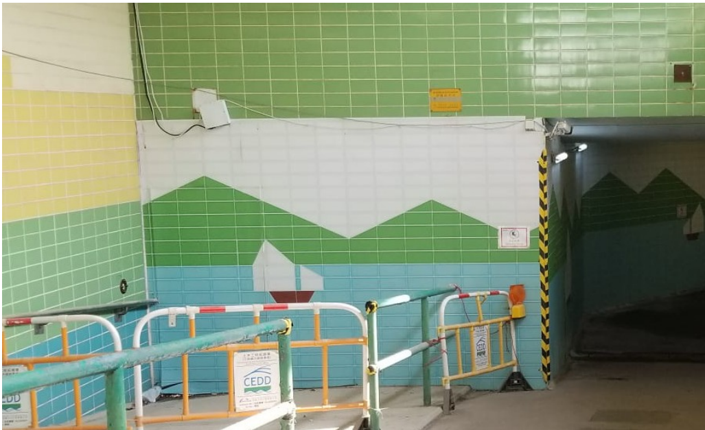
Photo 3 – Erection of site hoardings in unobtrusive colours
