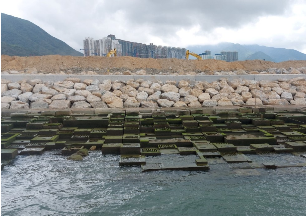
Photo 4 – Natural Rock Material/Planting for Artificial Seawall
