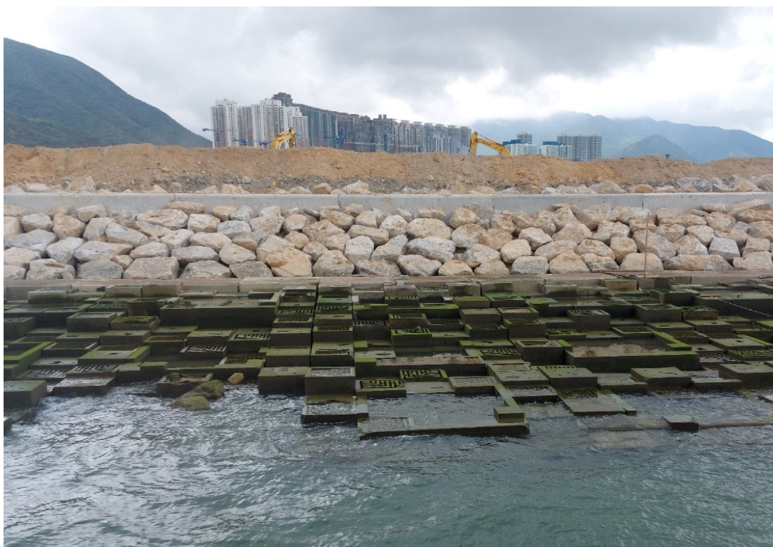
Photo 4 – Natural Rock Material/Planting for Artificial Seawall
