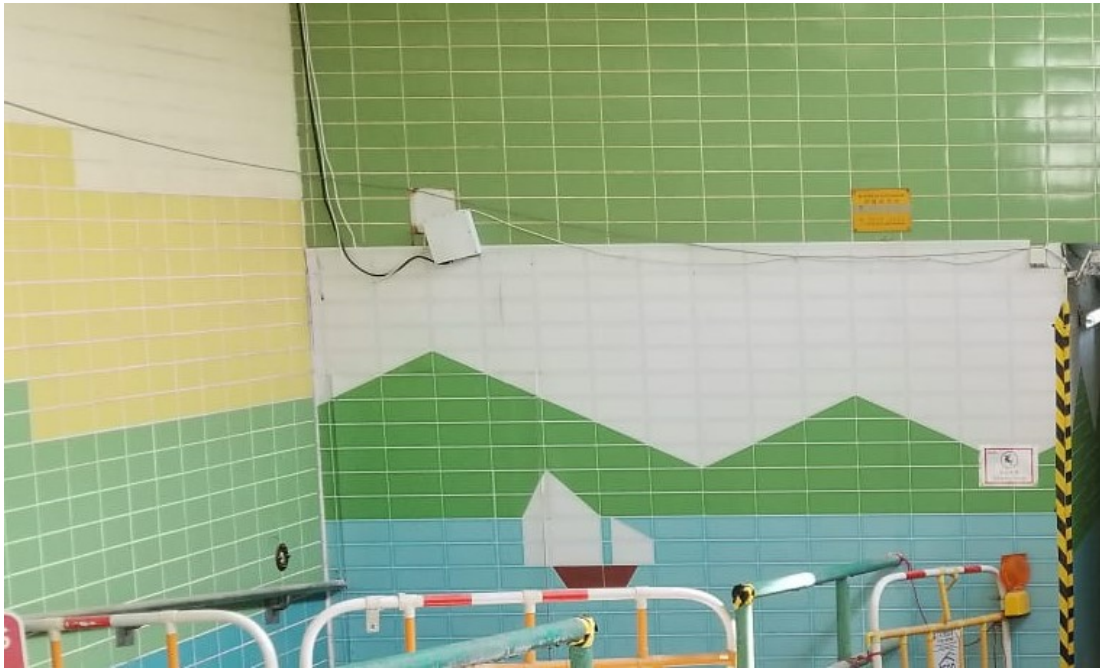
Photo 3 - Erection of site hoardings in unobtrusive colours
