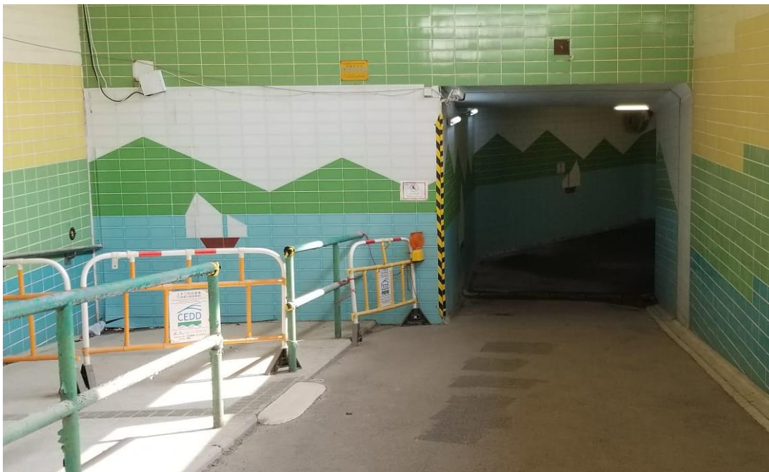
Photo 3 - Erection of site hoardings in unobtrusive colours
