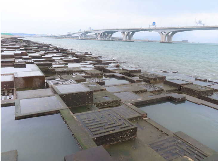
General View of Rocky Eco-shoreline
