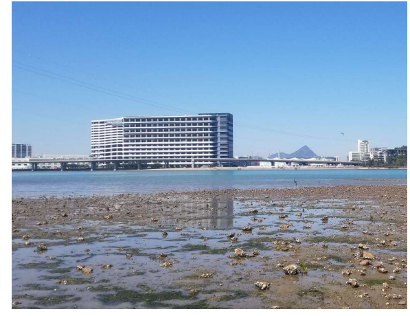
(c) Survey Location at TCB3
