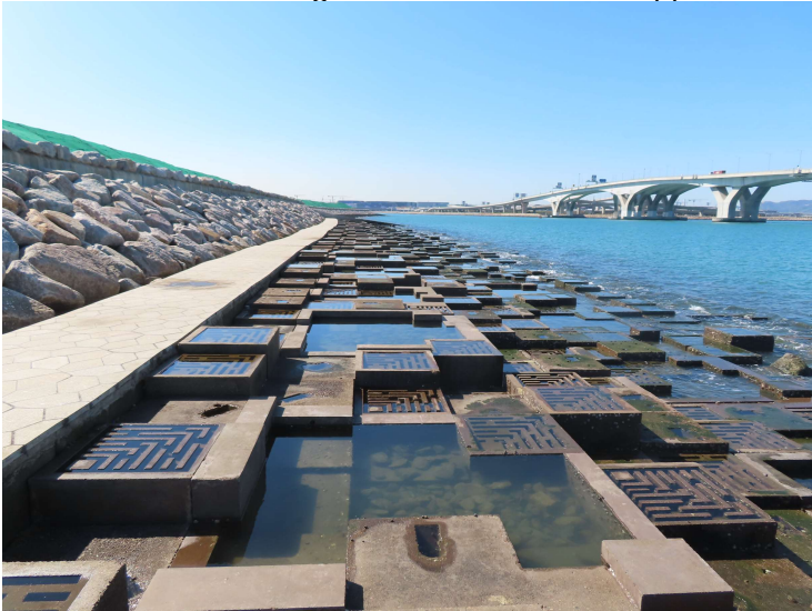
General View of Rocky Eco-shoreline
