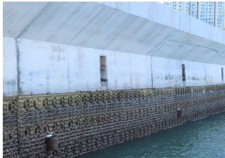
General View of Vertical Eco-shoreline
