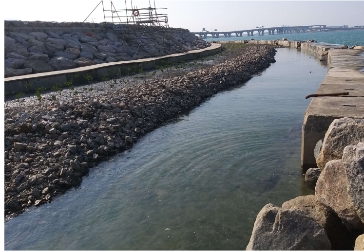
General View of Mangrove Eco-shoreline at Lower Terrace
