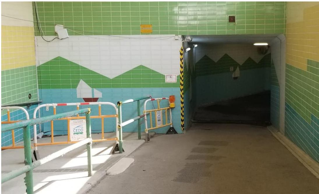
Photo 3 – Erection of site hoardings in unobtrusive colours
