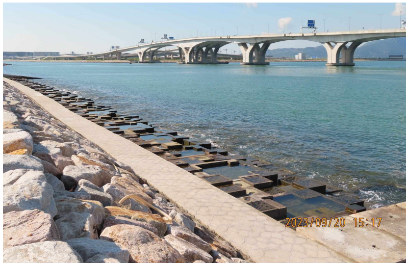
General View of Rocky Eco-shoreline
