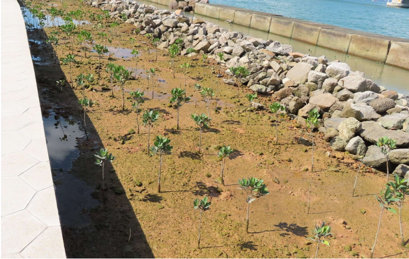
General View of Mangrove Eco-shoreline Upper Terrace
