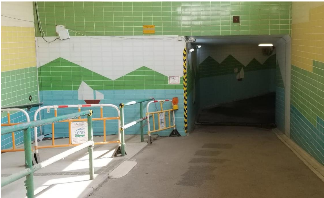
Photo 3 – Erection of site hoardings in unobtrusive colours
