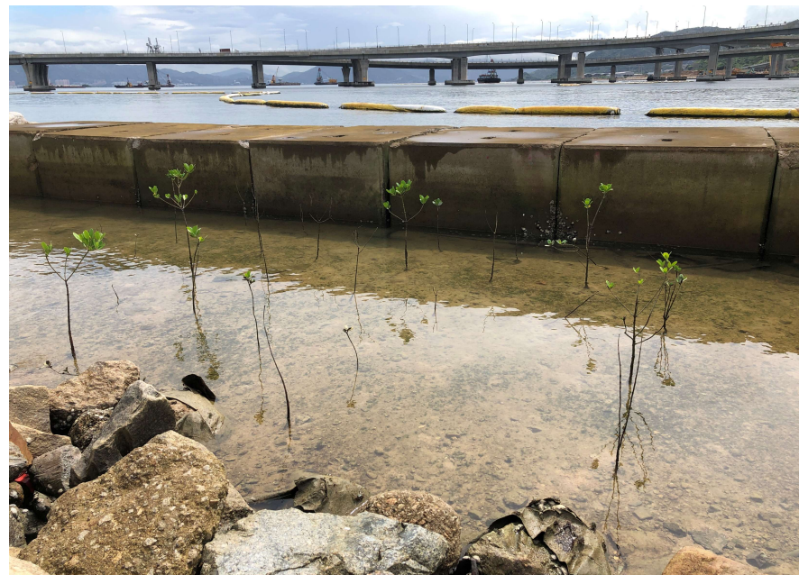
General View of Mangrove Eco-shoreline Lower Terrace
