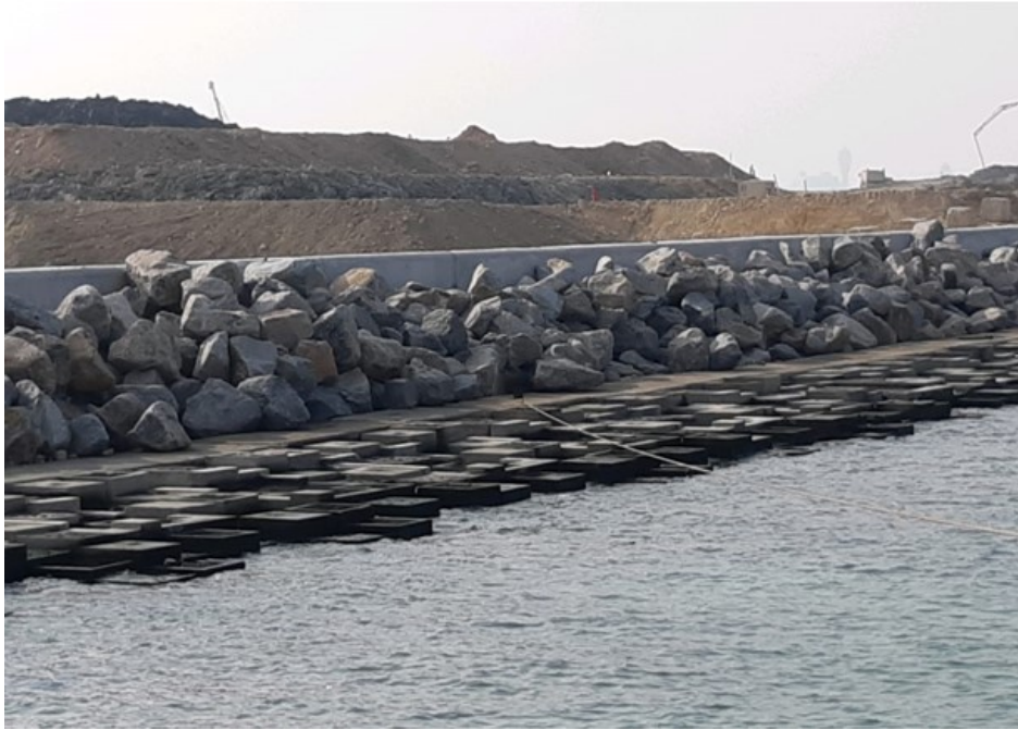
Photo 3 - Natural Rock Material/ Planting for Artificial Seawall
