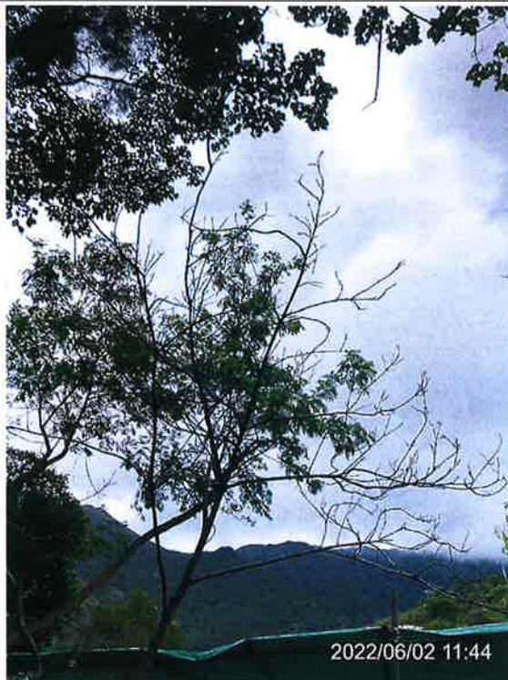
Photo 07: Crown condition of G62/RT-08
