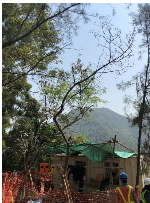
Photo 04: Whole view of G62/RT-07
