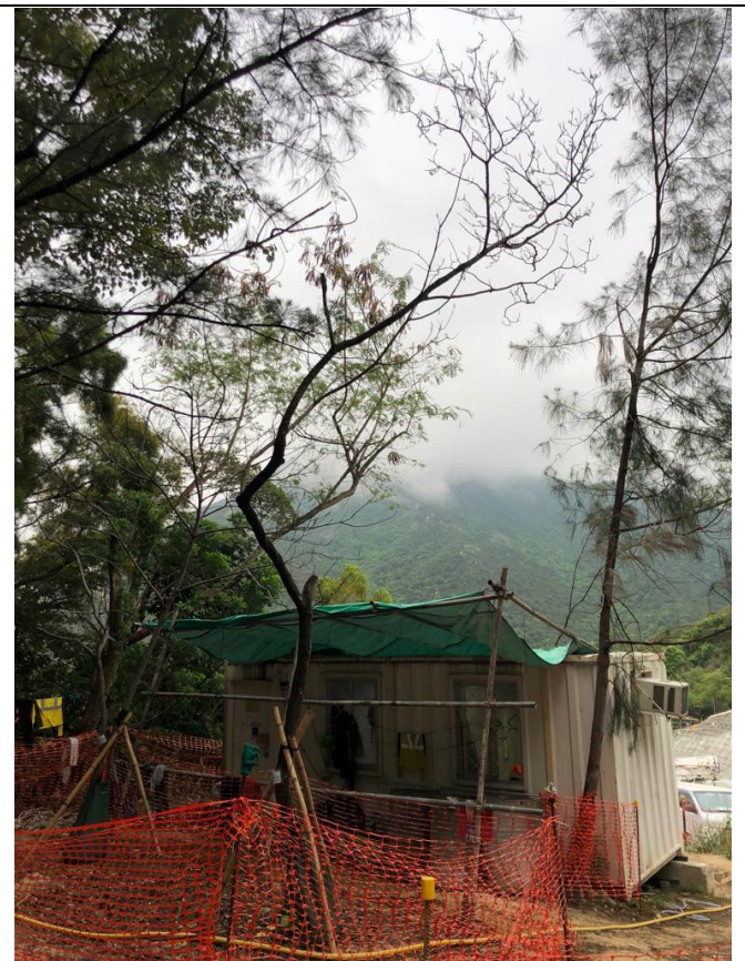
Photo 04: Whole view of G62/RT-07
