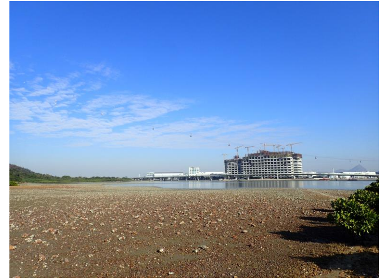
(c) Survey Location at TCB3
